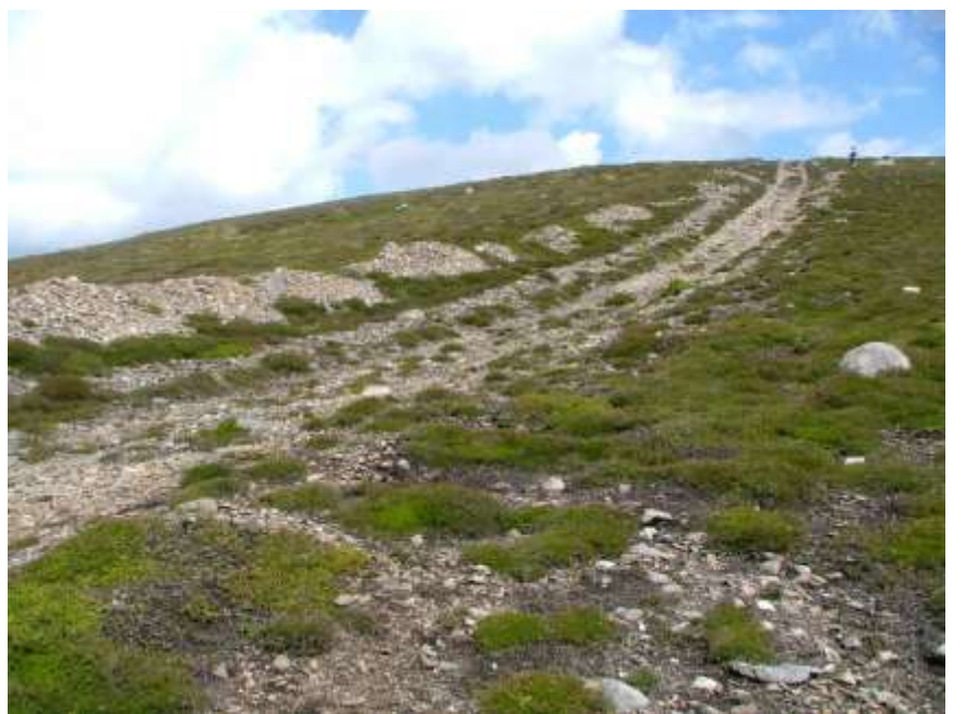
Above: Crudely engineered track near Ballater
