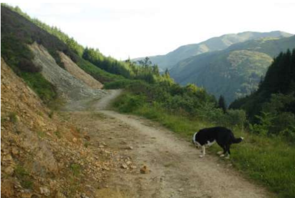
Below: Eroding forestry track, Glen Ample
