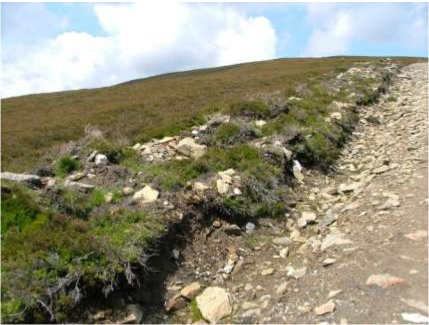
Below: Damaged verges on track near Ballater
